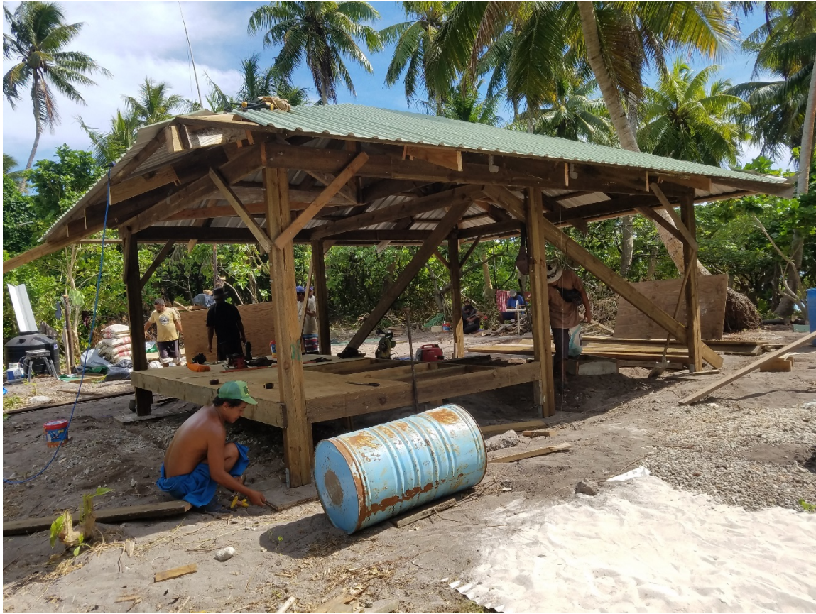
Figure 4-6 Progress on the camp structure on Loosiep Island. The final camp has an additional roofed section, an enclosed secure storage section, and a separate cooking unit, also two water catchments installed to collect water (final image n/a at time of writing).
